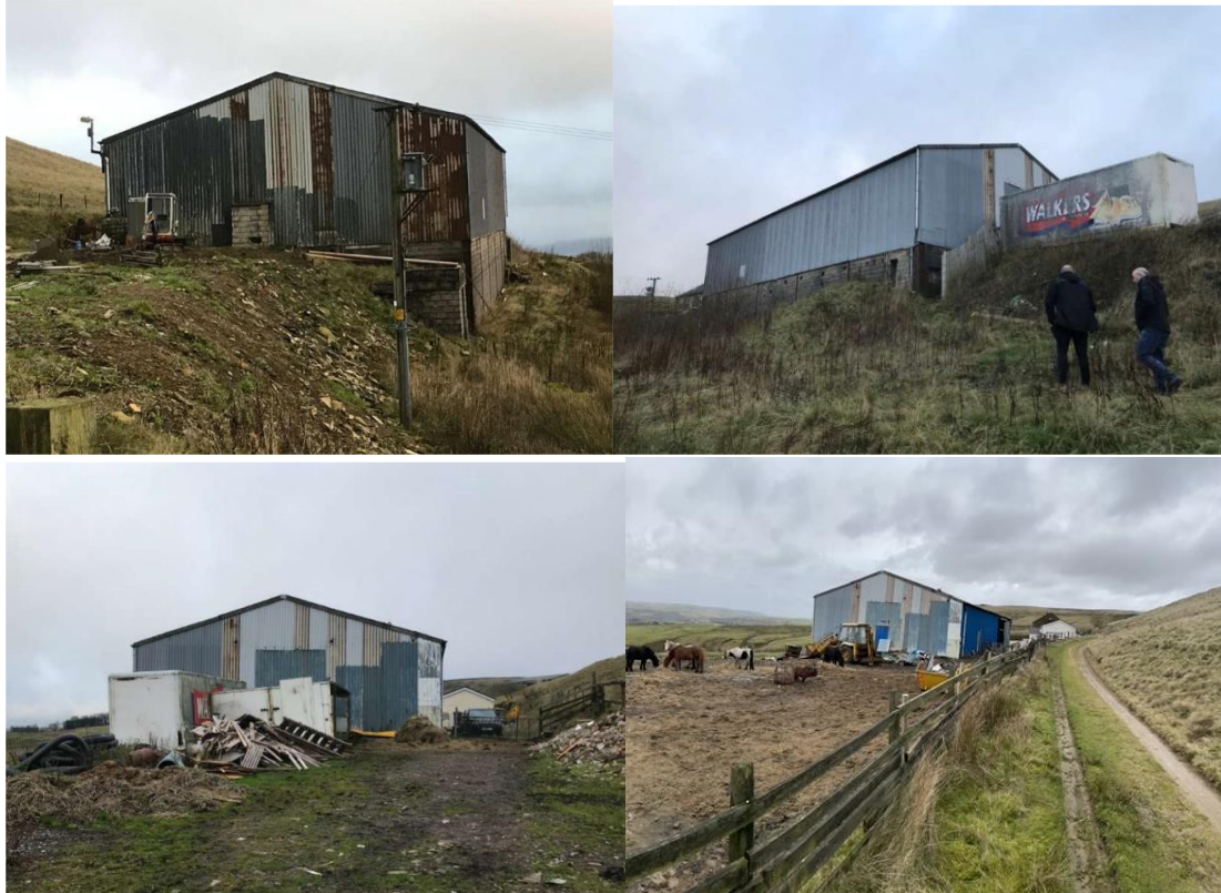
Fig 1: Images of existing barn structure
